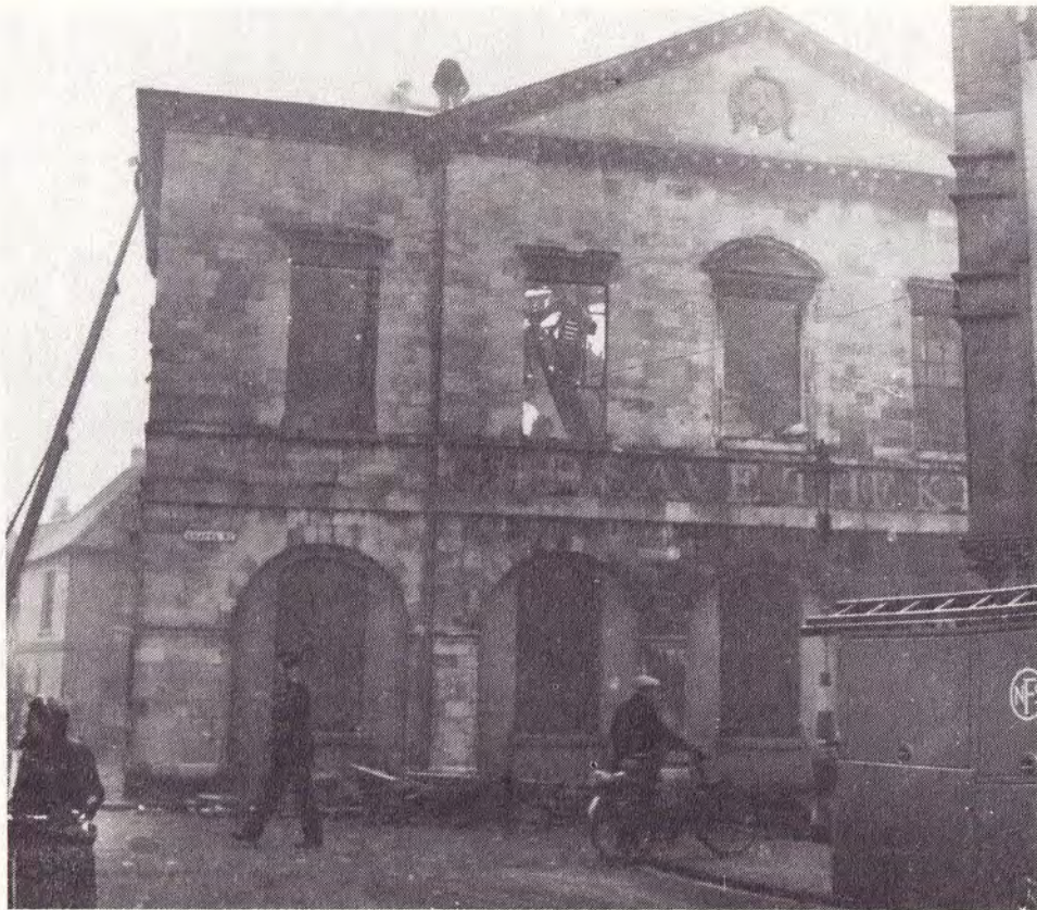
5 December 1946. Daylight revealed the full extent of the damage. The roof stairs can be seen collapsed into the ballroom.
