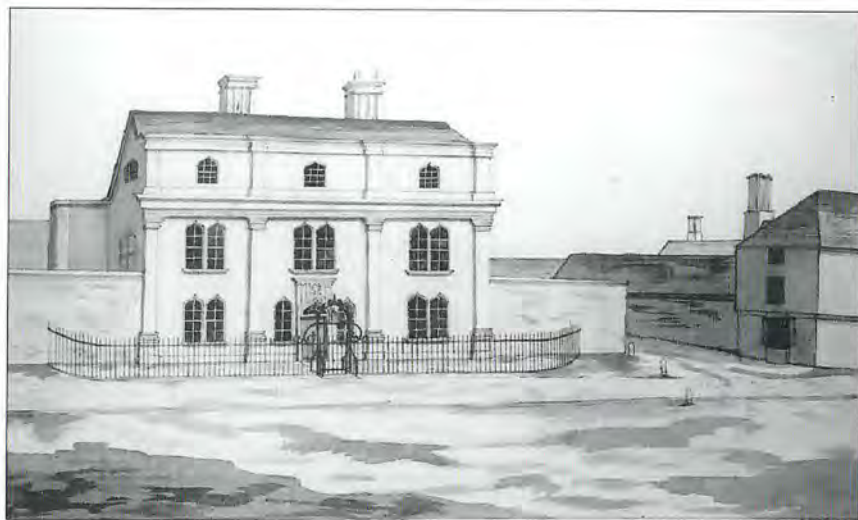
46. No. 16 Church Street, after its first re-fronting in 1768, when Gothic windows and pilasters appeared. During the second facelift (1840) the Gothic windows survived but the pilasters were removed or covered over and the present battlements added.
