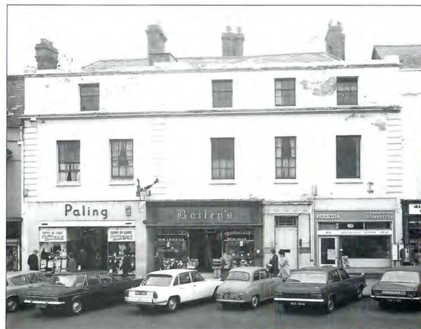
4. No. 11 Bridge Street, c. 1970. Only the front wall was left standing, and the front door moved to a 'more convenient' position, when this building was converted to a Boots store.
