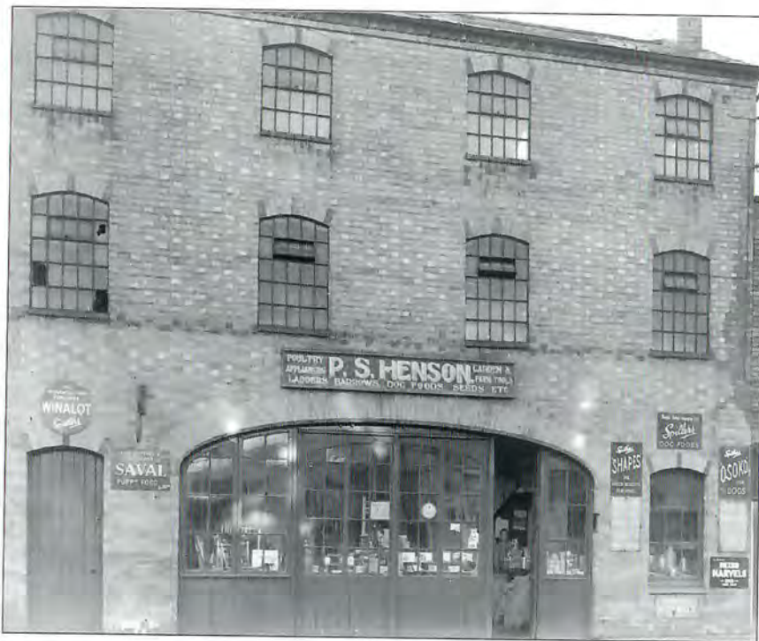
34. No. 25 Greenhill Street in the 1930s, with its wide arched entrance still a prominent feature.
