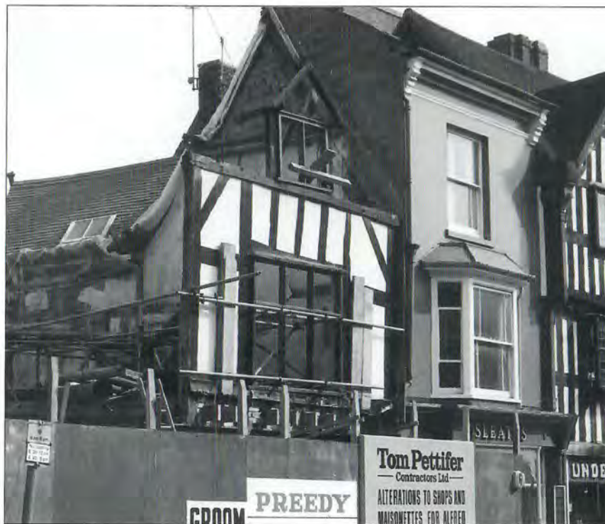
15. Only the front wall of No.15 was left standing during 1977 redevelopment work and No. 14 was completely demolished and rebuilt.
