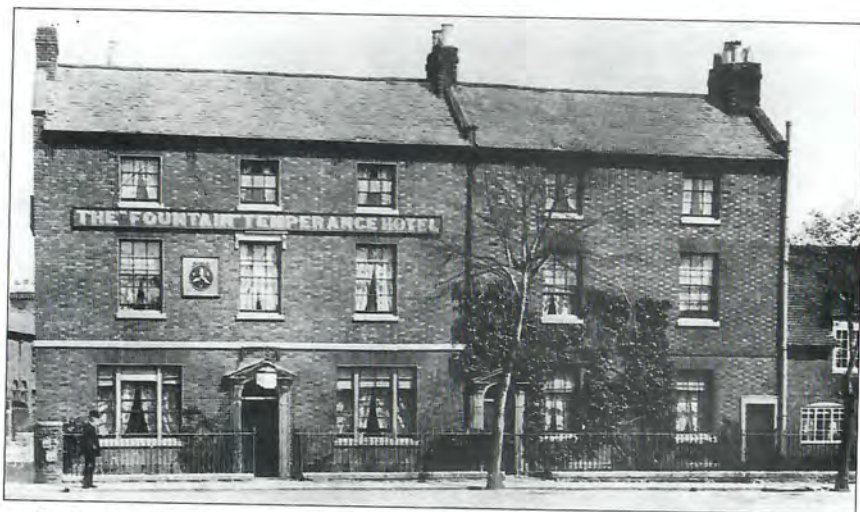
29. Nos. 20-21 Rother Street, on the corner of Windsor Street, c. 1910. The character of these handsome houses, dating from around 1810, has been undermined by the addition of obtrusive and unsuitable shop fronts.
