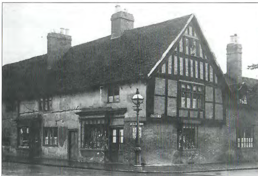
9. No. 26/27/28 Wood Street, c. 1915. Its old timber-frame was then partly concealed by early nineteenth-century stucco.
