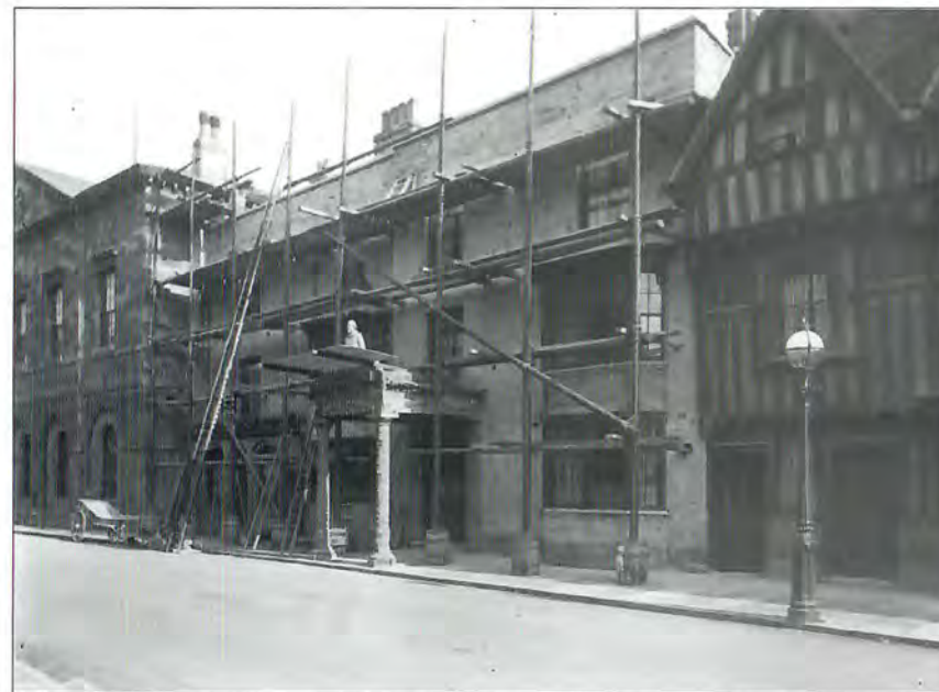
26. Rebuilding the front wall of the Shakespeare Hotel, 1920. The portico was salvaged and attached to the Red Horse in Bridge Street.
