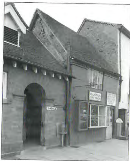
28. No. 34 Rother Street in the early 1970s. Its timber-frame, concealed by a brick skin, only became obvious when the public conveniences next door were demolished to form an entrance into the multi-storey car park.
