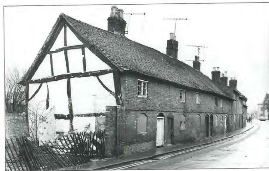
39. Nos. 30-34 Ely Street, timber-framed cottages with their front walls rebuilt in brick in the early nineteenth century. During restoration in the 1970s, timber-framing was re-instated along the street but in an ill-informed manner.
