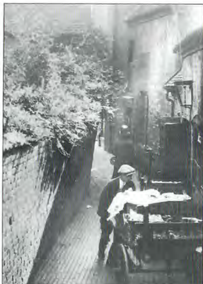
19. Cooks Alley, linking Wood Street and Henley Street, before widening in the mid 1930s.
