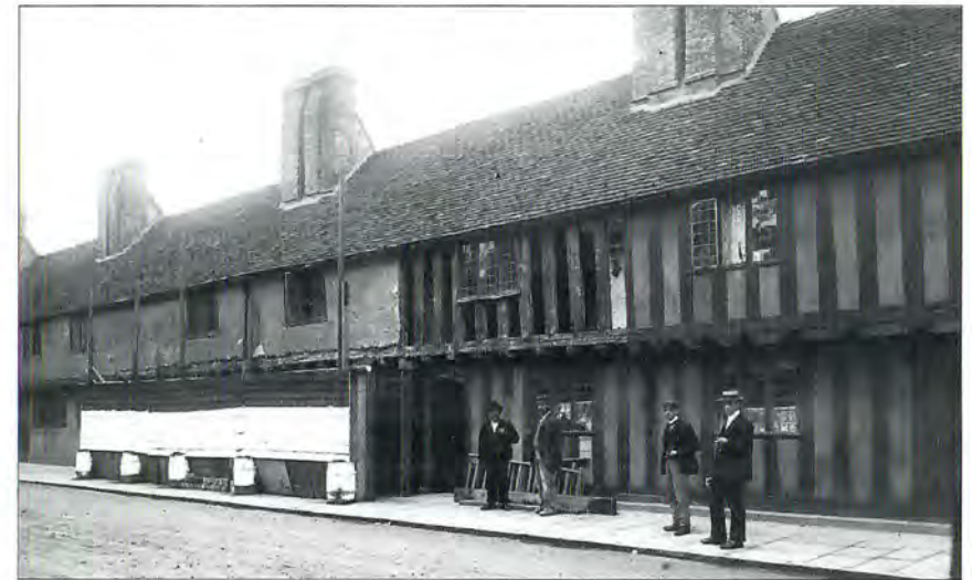
45. Early nineteenth-century stucco being removed from the original timber-framing of the almshouses in Church Street during restoration in 1902-03.
