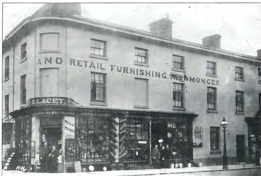
12. No. 1 Wood Street, c. 1900. This was given a stucco finish when built in 1840 to match similar buildings in nearby Bridge Street.
