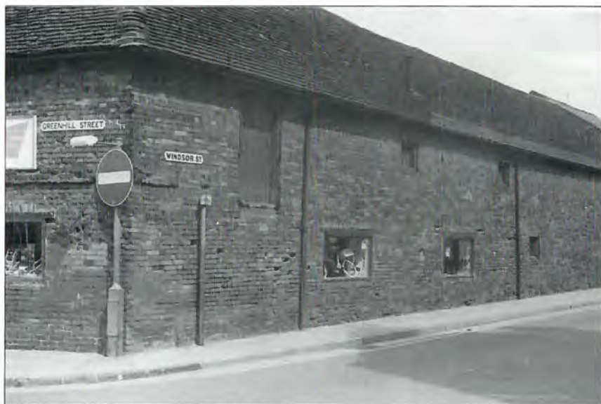
32. No. 22 Greenhill Street, originally a barn, partially rebuilt around 1800, and still retaining much its character in this 1969 photograph.
