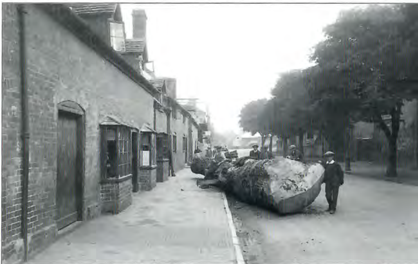
41. Eighteen cottages, which stood in Waterside between Bridge Street and Sheep Street, were demolished in stages from 1913. This photograph, from 1914, reminds us that until the 1930s, those living here did not look out across well-maintained gardens but were faced from across the road with warehouses built around the canal basin.
