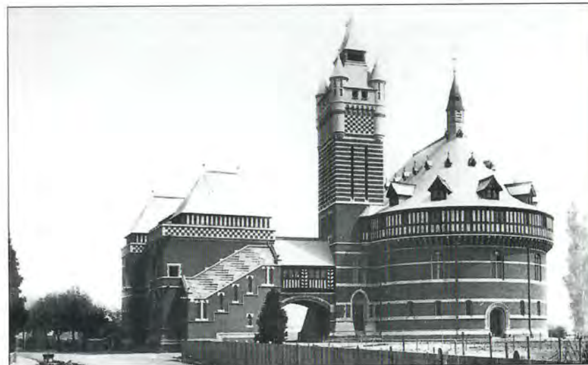
54. The Shakespeare Memorial Theatre soon after the completion of building works in 1881, an extraordinary building designed by Edward Dodgshun and William Unsworth. Following the fire in 1926, the tower was demolished and the remains of the original roof removed. The picture gallery on the left survived as did the shell of the old auditorium on the right. In 1985 this was re-roofed and converted into the Swan Theatre.
