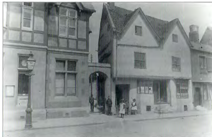
23. No. 42 Sheep Street, c. 1895, before a restoration which revealed its timber-frame. The building to its left was the Post Office, since demolished.
