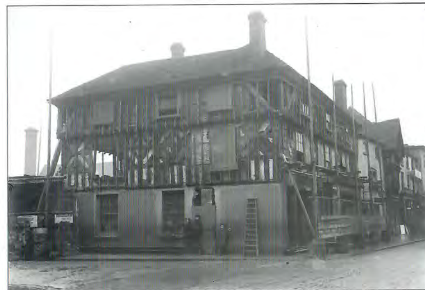
2. The timber-frame of No. 23/24 High Street (on the corner of Ely Street) emerging from behind its stucco facing during restoration in 1903.
