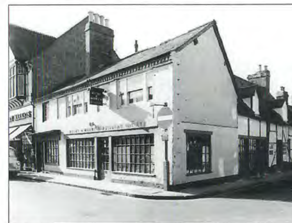
17. No. 53 Henley Street in 1970, a timber-framed building refronted in about 1800. A severe 'restoration' has since transformed its appearance for the second time.
