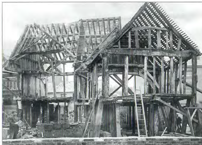
18. Rear view of the Public Library in Henley Street, at mid point in its 1904 restoration.
