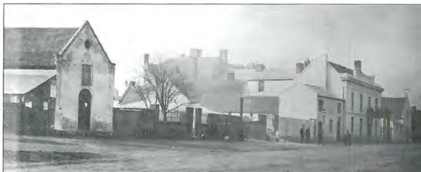
58. Guild Street around 1850 before the improvement scheme narrowed it to its present width.
