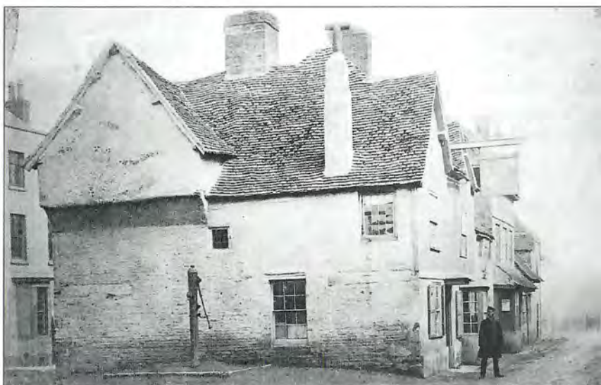
3. The last remaining houses in Middle Row, Bridge Street, demolished in the late 1850s.
