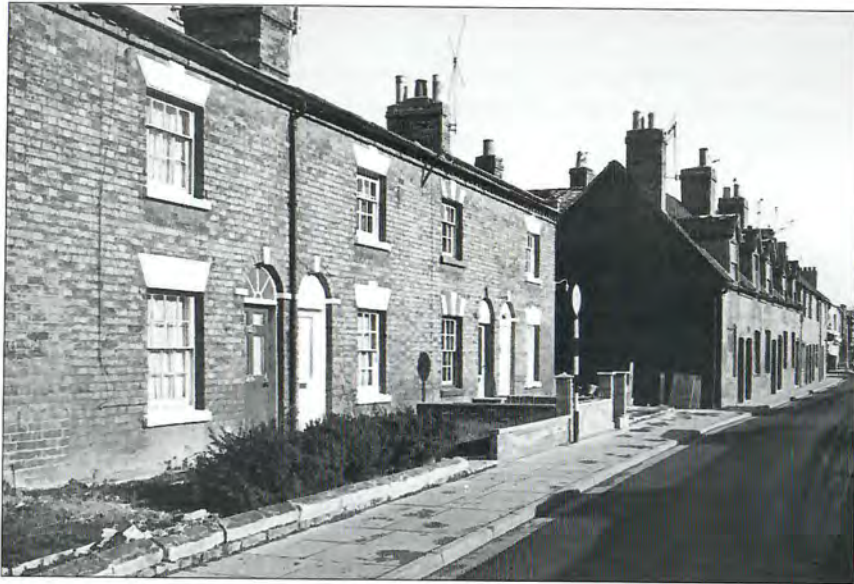
35. The west side of Windsor Street, before the demolitions of the 1960s. Both these terraces have now disappeared, seriously compromising the street's residential character
