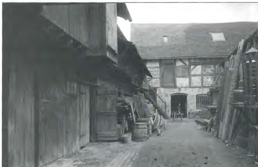
40. This courtyard to the rear of Nos. 59-60 Ely Street was typical of the many semi-open spaces behind the street frontages. Many have since been built over but this one still survives.
