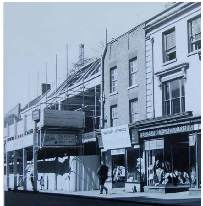
Fig. 4: Demolition of Nos 33/4 and 35 High St., c.1960
