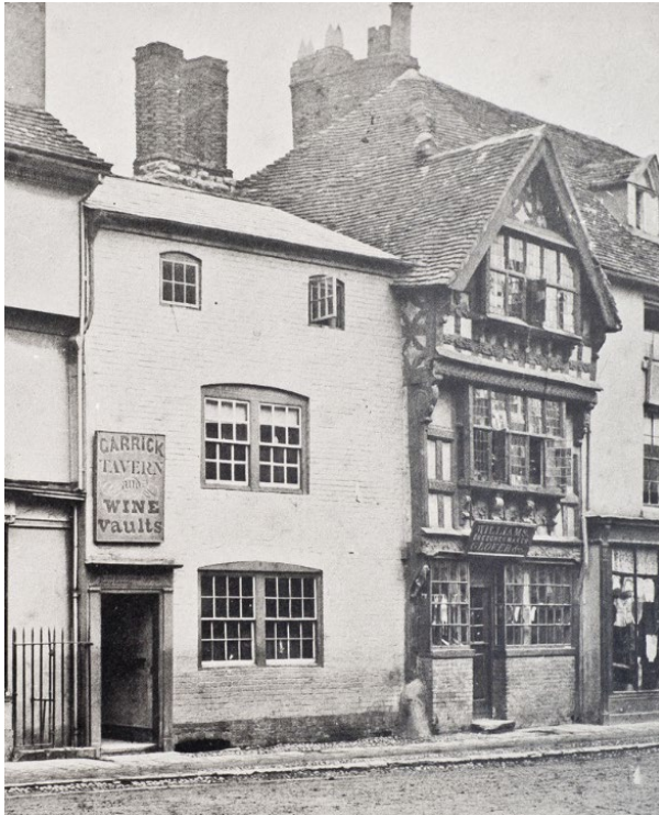
Fig 2: Garrick Inn, c. 1895, re-fronted in brick earlier in that century
