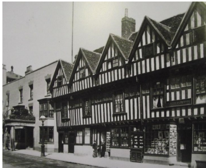
Fig. 3: Photograph from c.1895 with the plaster removed
