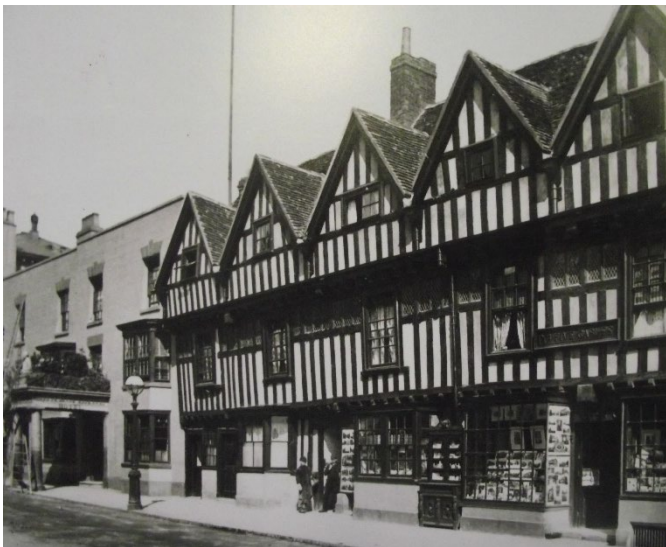
Fig 3: photograph from c. 1895 with the plaster removed
