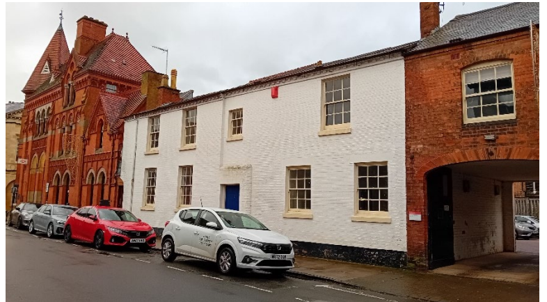
Fig. 7 Site of 1 Ely St, 2023
