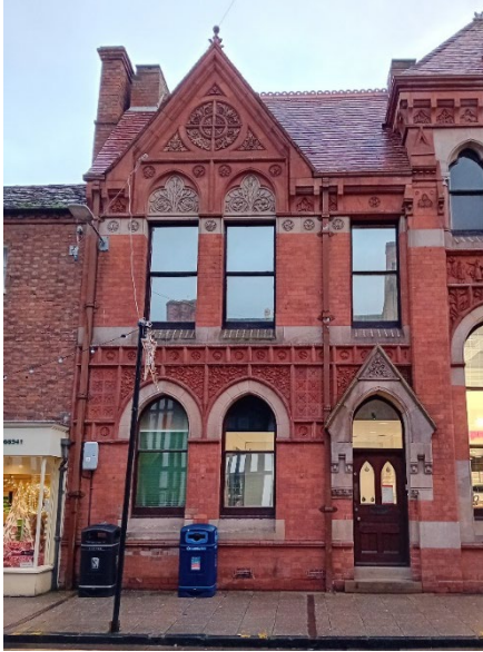
Fig 1. site of No. 12 Chapel St, 2023
