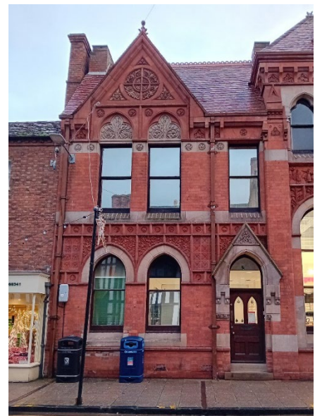
Fig. 4: site of No. 12 Chapel St, 2023.
