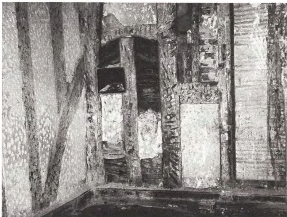
(b) Original doorway in south-east corner of Big School, discovered behind the plaster in 1949 (Reproduced by courtesy of T. F. Holte, Esq., Stratford-upon-Avon)
