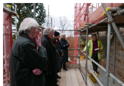
North transept of church
