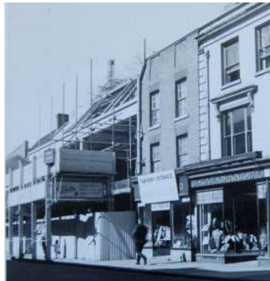
Fig 2: Demolition of Nos 33/4 and 35 High St, c. 1960
