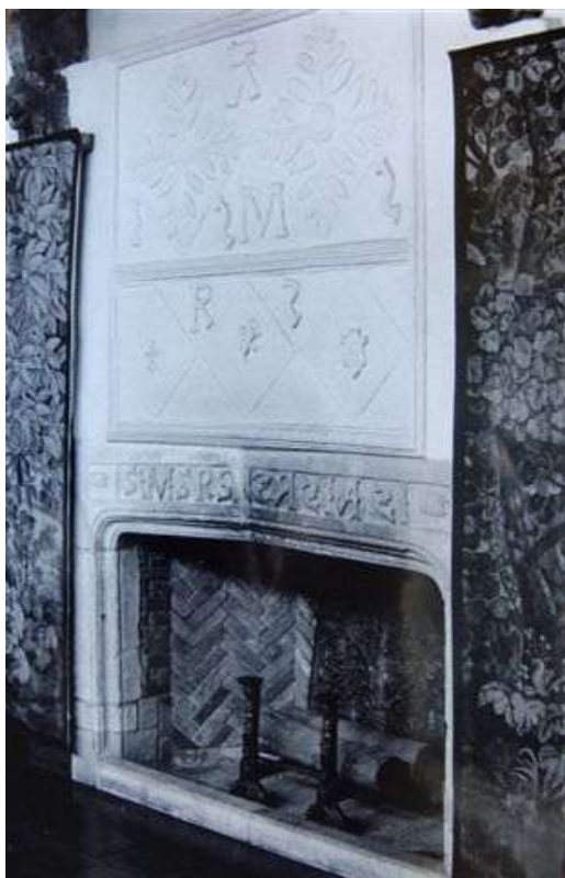
Fig. 3: The 'Stratford' fireplace at Packwood House, salvaged from No. 35 High St
