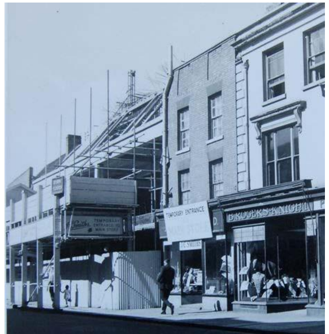
Fig 4 : Demolition of Nos 33/4 and 35 High St, c. 1960
