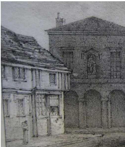
Fig 3: Town Hall and No. 22 High St, 1810
