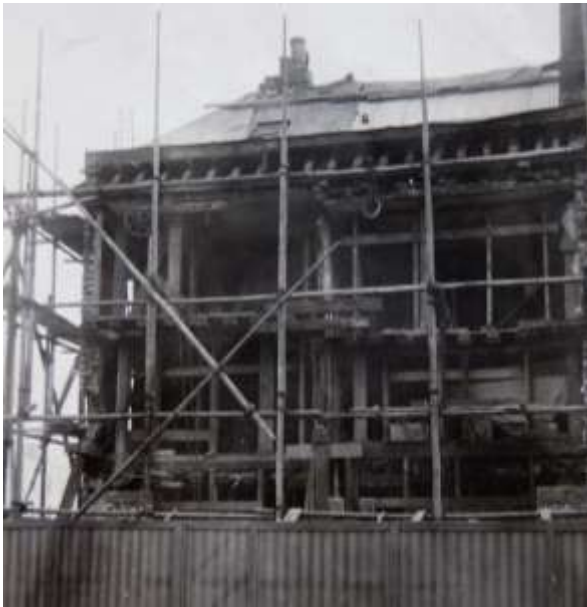
Fig.3: internal framing exposed during restoration of 1923.
