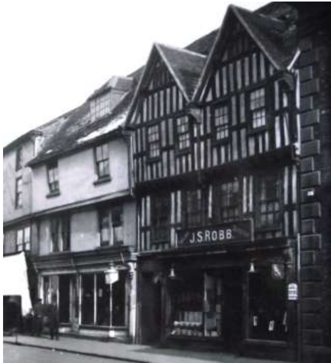
Fig. 7: The stucco was removed from No. 21 in 1913
