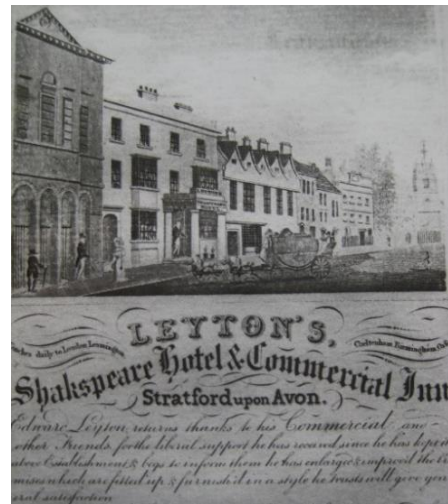
Fig. 4. Trade card from the 1830s showing the new frontage to the Shakespeare Hotel
