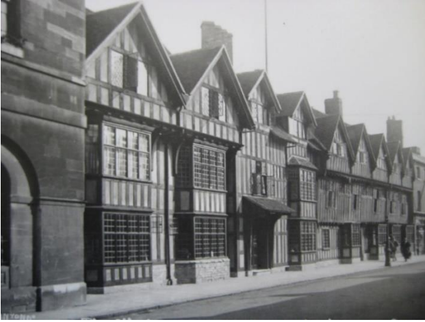
Fig. 7 Shakespeare Hotel, following restoration, 1920
