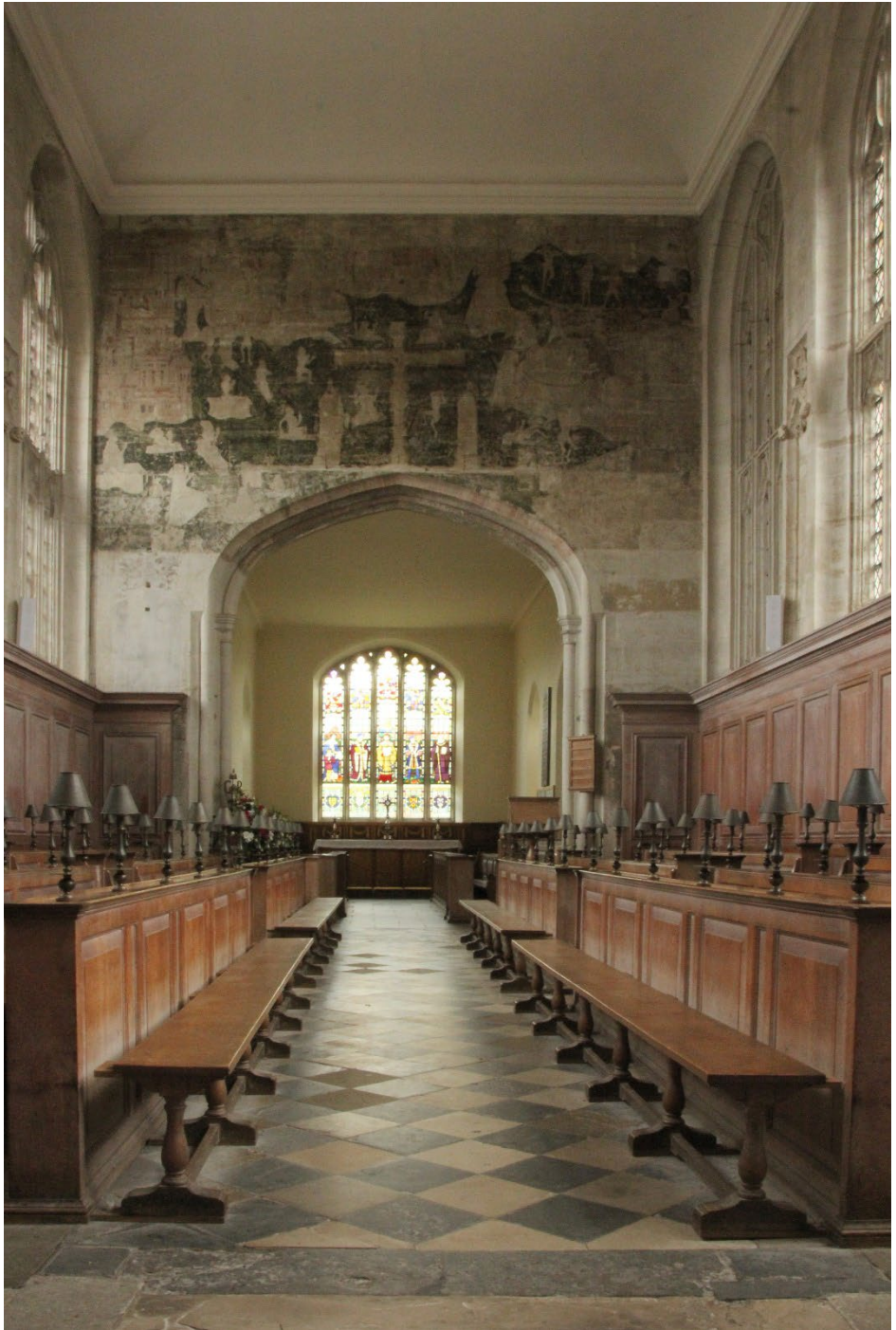
Interior of the Guild Chapel looking east, showing Doom painting above the arch.
