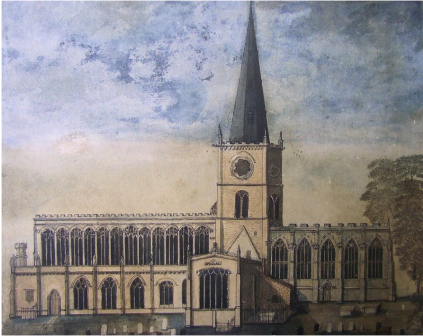
John Jordan's late 18th-century drawing of the south elevation of Holy Trinity Church, showing the south transept after the removal of its steeply-pitched 13th-century roof.
