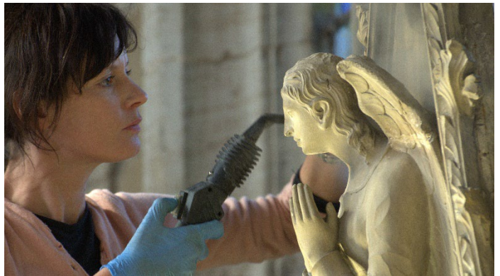
Cleaning the angel at the apex of the Davenport memorial, using a 'dry-steam' cleaner, which emits a jet of steam at 160°C.
