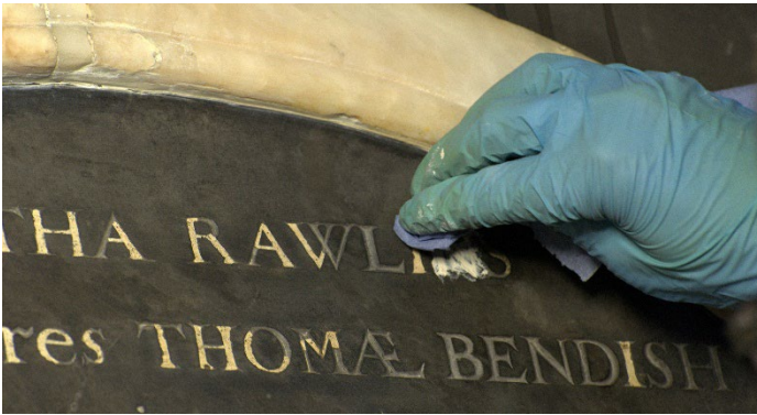
Filling the incised letters with a lime-based filler, which was then toned in with acrylic paints.
