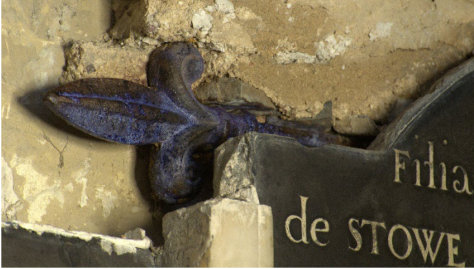
The fleur de lys support found incorporated in the Rawlings memorial, after treatment to inhibit rust.
