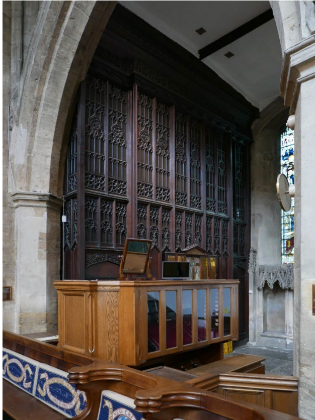
Oblique view from choir stalls of the organ console and the wooden oak screen designed by Messrs Bodley and Garner to conceal the organ.
