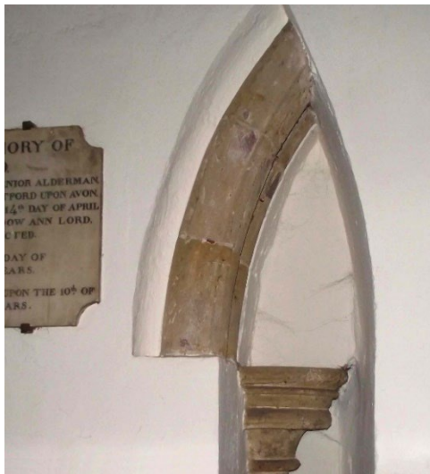
13 th century capital of the blocked arch leading from north transept to chancel aisle.
