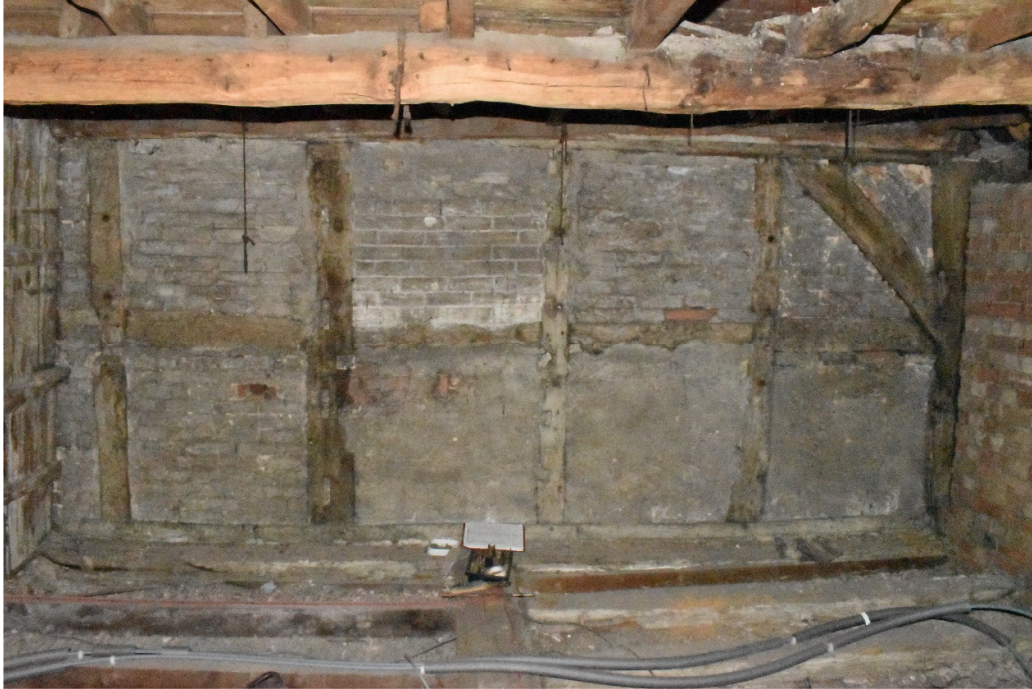
Plate 36: Unit B; large-panel framing of Bay Vc (west); see also Plate 00.
