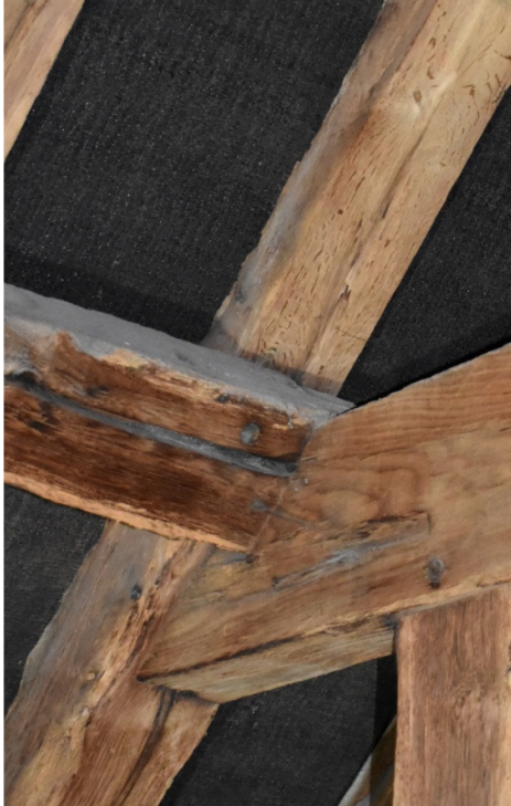
Plate 41: Unit B; detail of diminished principal at collar level, above clasped purlin (T11).
