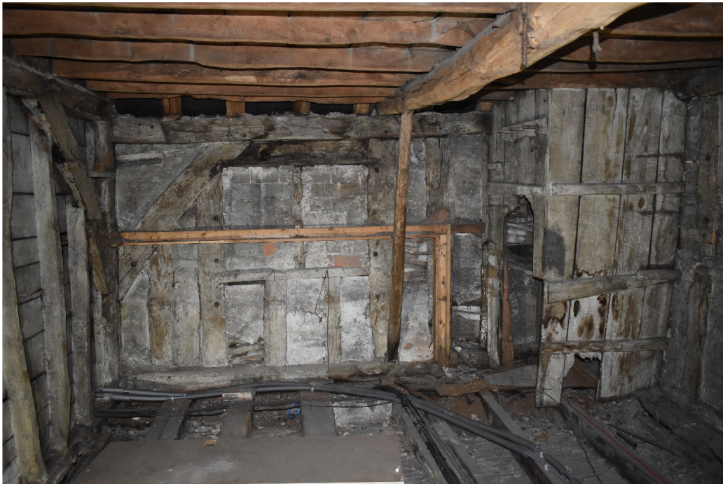
Plate 35: Unit B; detail of close-stud walling at Bay Vc (south) with blocked secondary window.
