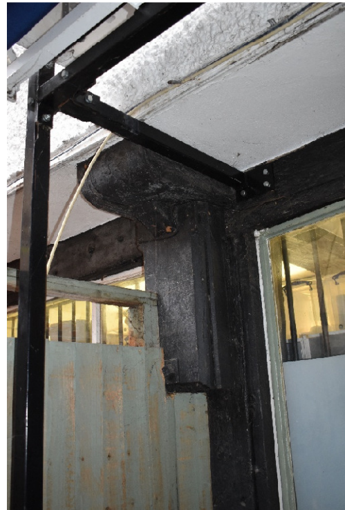
Plate 31: Unit B; detail of replacement bracket.
