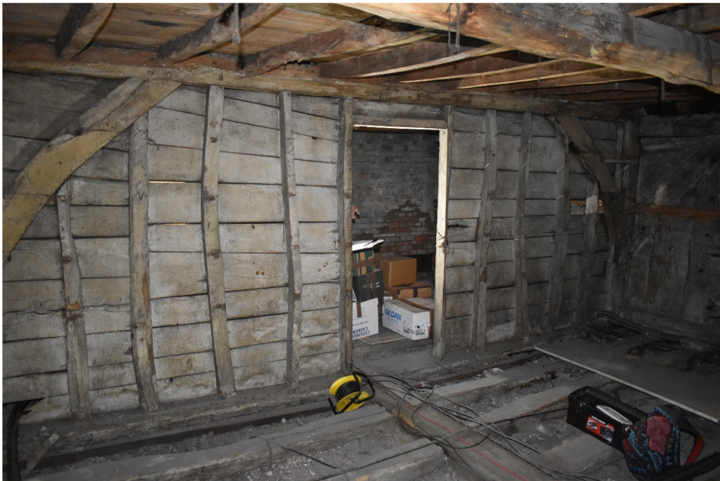
Plate 37: Unit B; boarded partition at Bay Vb/Vc, looking east.
