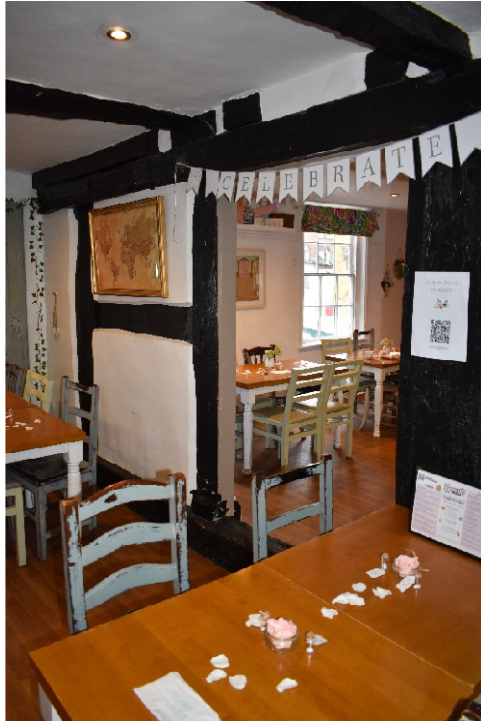
Plate 5: Unit A, Bay II; framed partition between [F6] and [F2] (inserted door).
