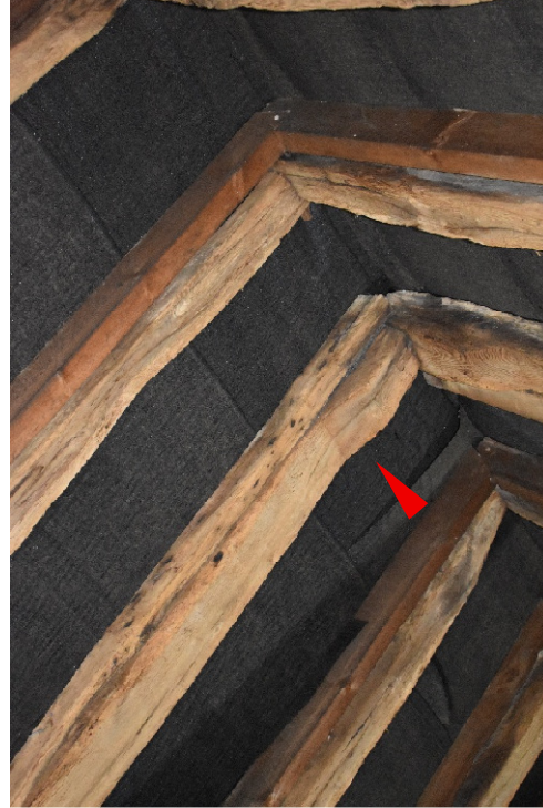
Plate 42: Unit B; detail of splayed principal at apex level (T11).
