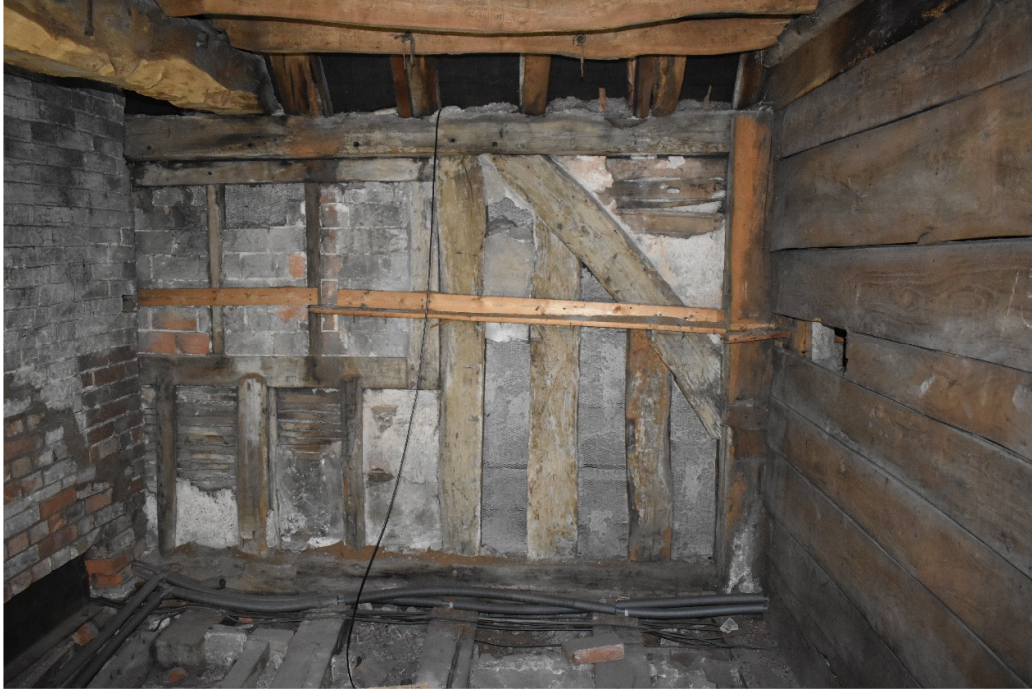
Plate 34: Unit B; detail of close-stud walling at Bay Vb (south) with blocked secondary window.
