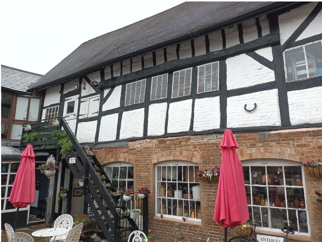
Plate 48: Unit C, Bay VIIb, yard elevation; note lower wall plate.
