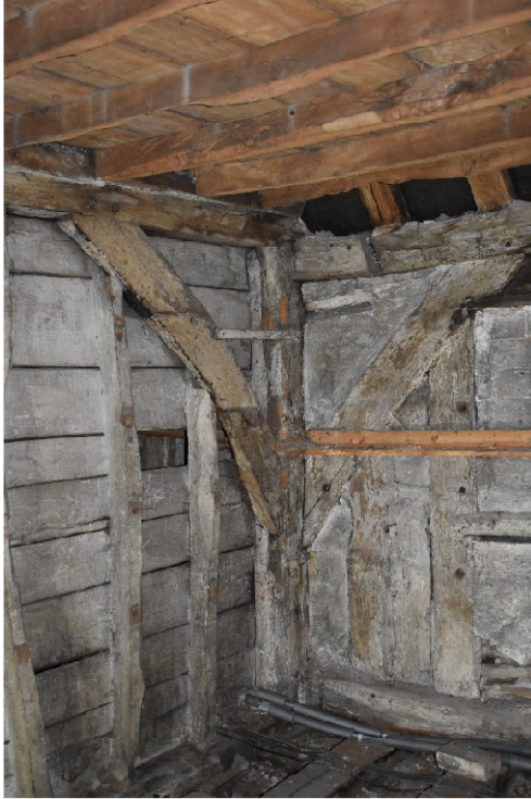
Plate 38: Unit B, bracing beneath T10(S).
