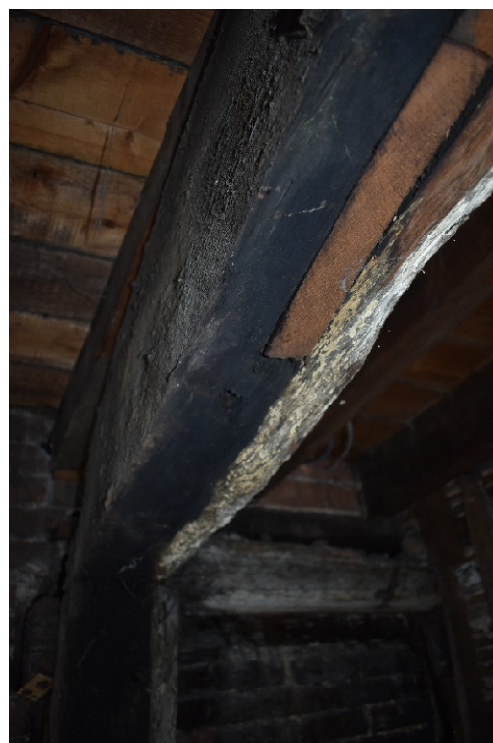
Plate 11: Unit A, Bay IV; heavy soot blackening to tie beam of truss T7a; NB. brace mortice.
